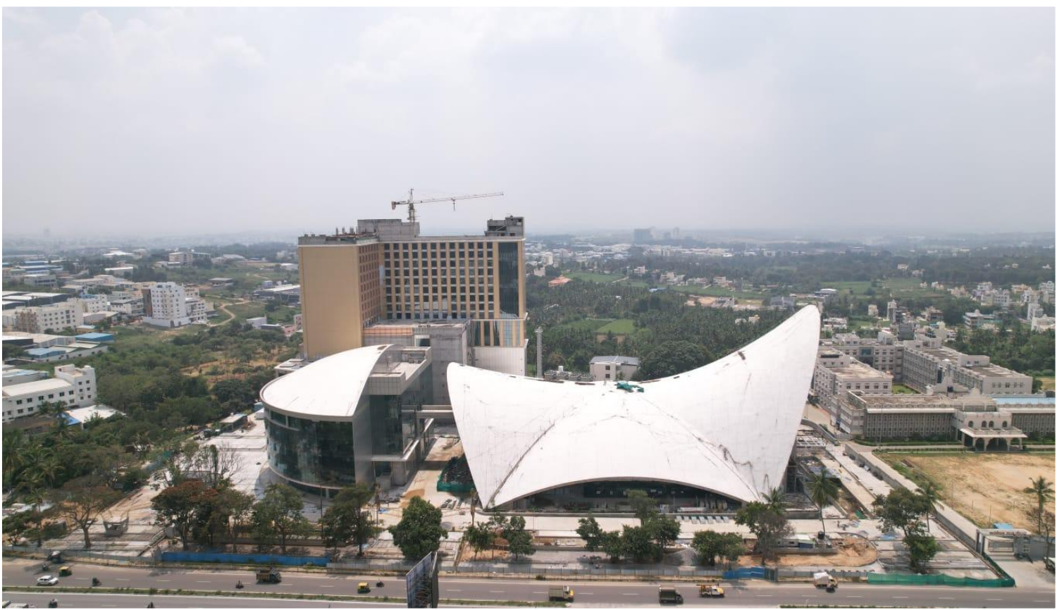
Jana Seva Trust Param, Bangalore (Work in Progress)
